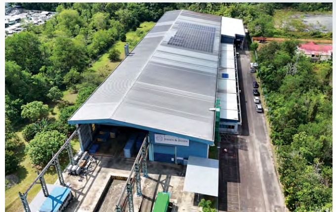
Solar PV system at MHE Johor Bahru facility.
